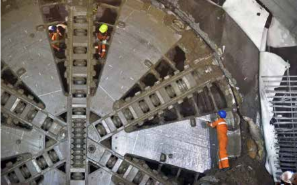
TBM cutter-head inspection
