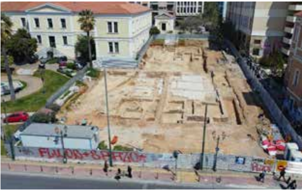
Akademia Station preparatory works
